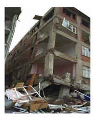
Figure 1. Seismic-induced damage of beam-column joints
