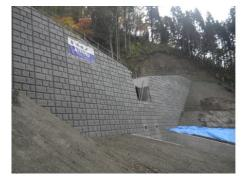
Figure 1 Sabo dam using soil-cement
